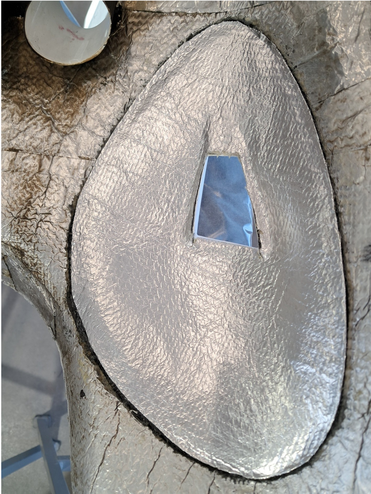
Fig. 21 Bonding of thermal insulation
