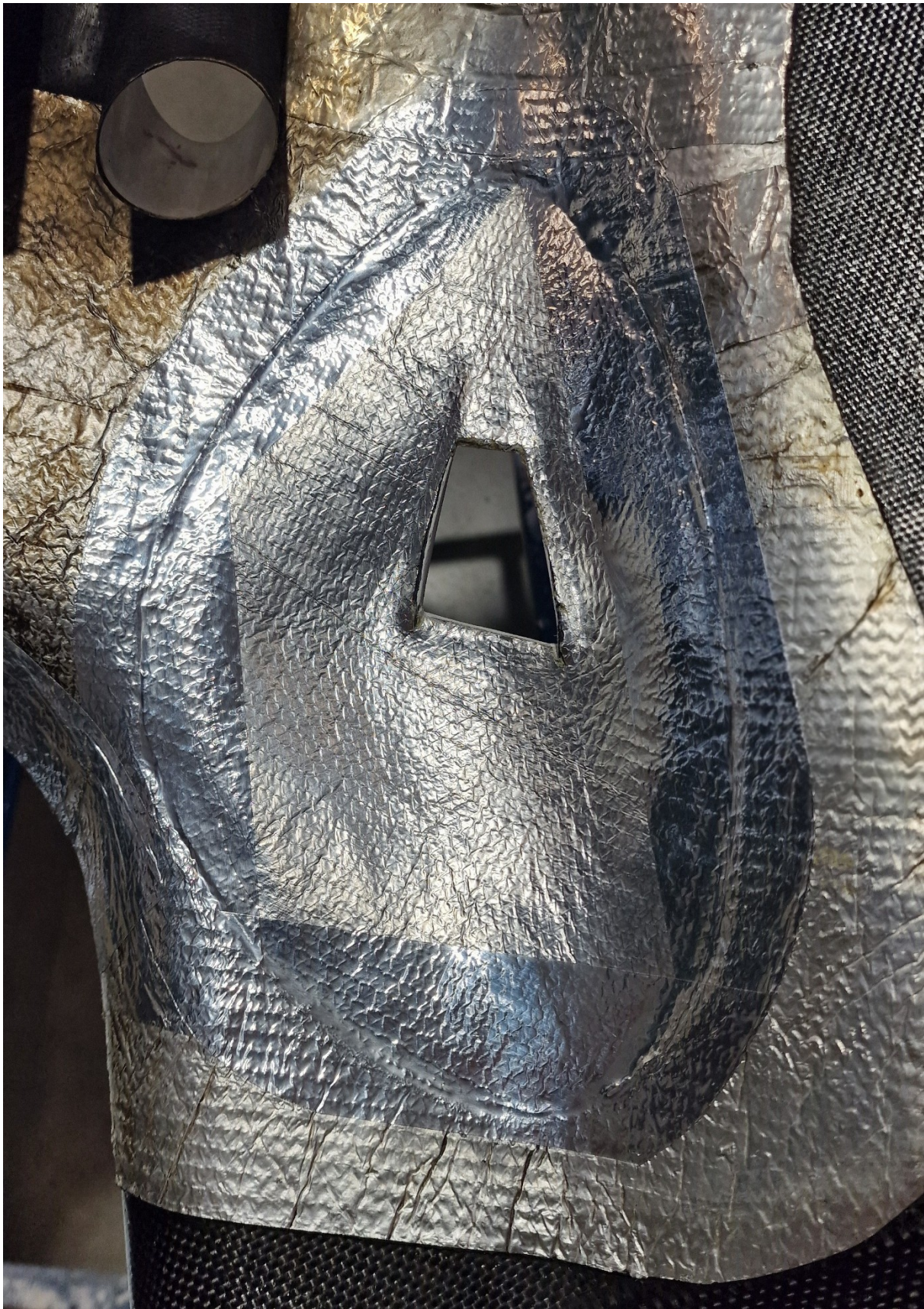
Fig. 22 Covering of thermal insulations joint
